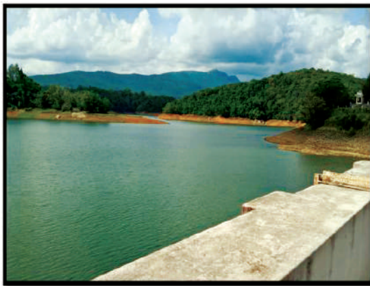
Fig. 1. Highland area (Neyyar Reservoir)
