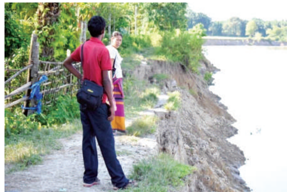
Fig. 13. Soil erosion on the bank of the Burhidihing river
